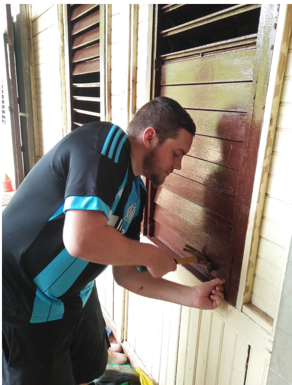
Matthieu installing the newly repaired and painted windows.
