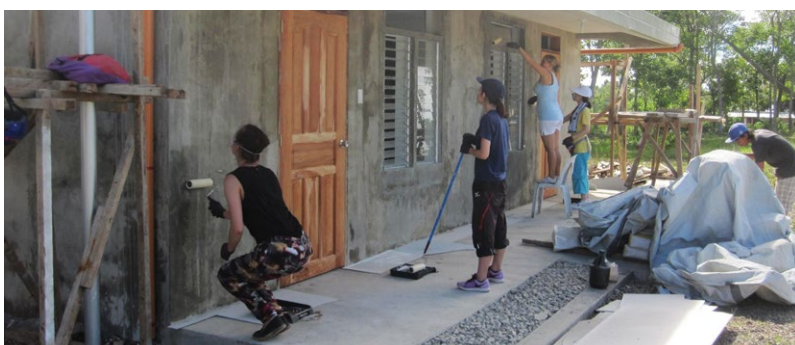
Volunteers applying a neutralizing agent, to take off the chemicals present in the cement that could affect the paint.
