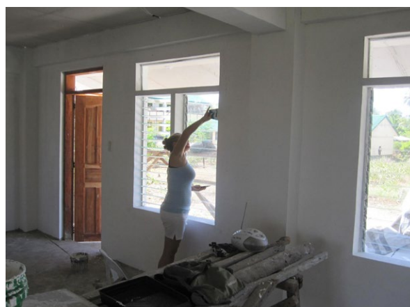
A volunteer applies a patching compound to cover the cracks of the wall.
