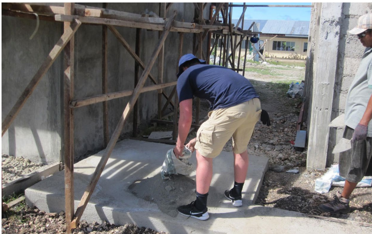
A volunteer mixing sand, cement and gravel in preparation for his assigned masonry work, behind the school building.
